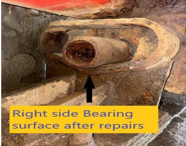
Barge Ramp Transition Repairs
