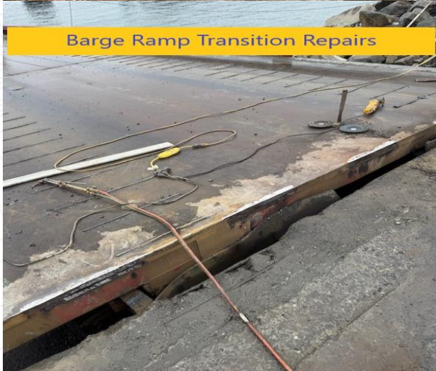
Right side Bearing surface after repairs
