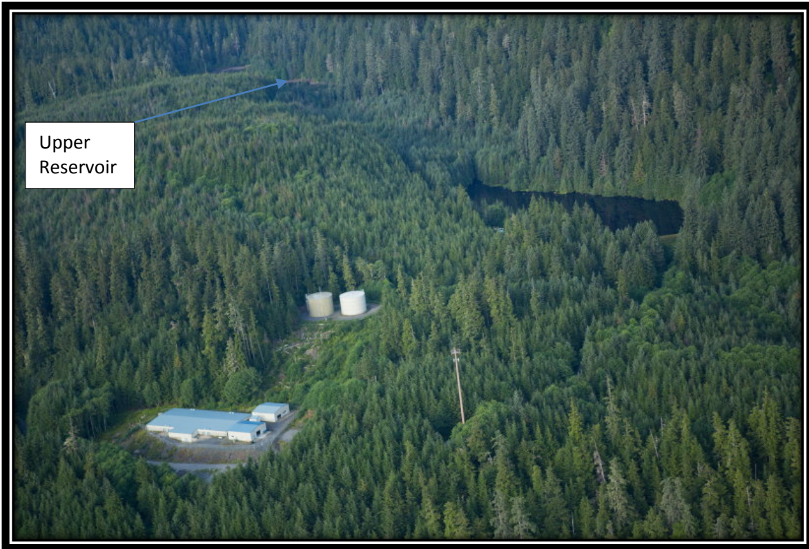
Water Treatment Facility
