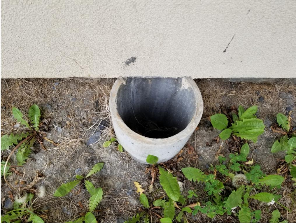
**Photo 11:** The cement standpipe near the southeast corner of the building is ACM. (May 23, 2018)
