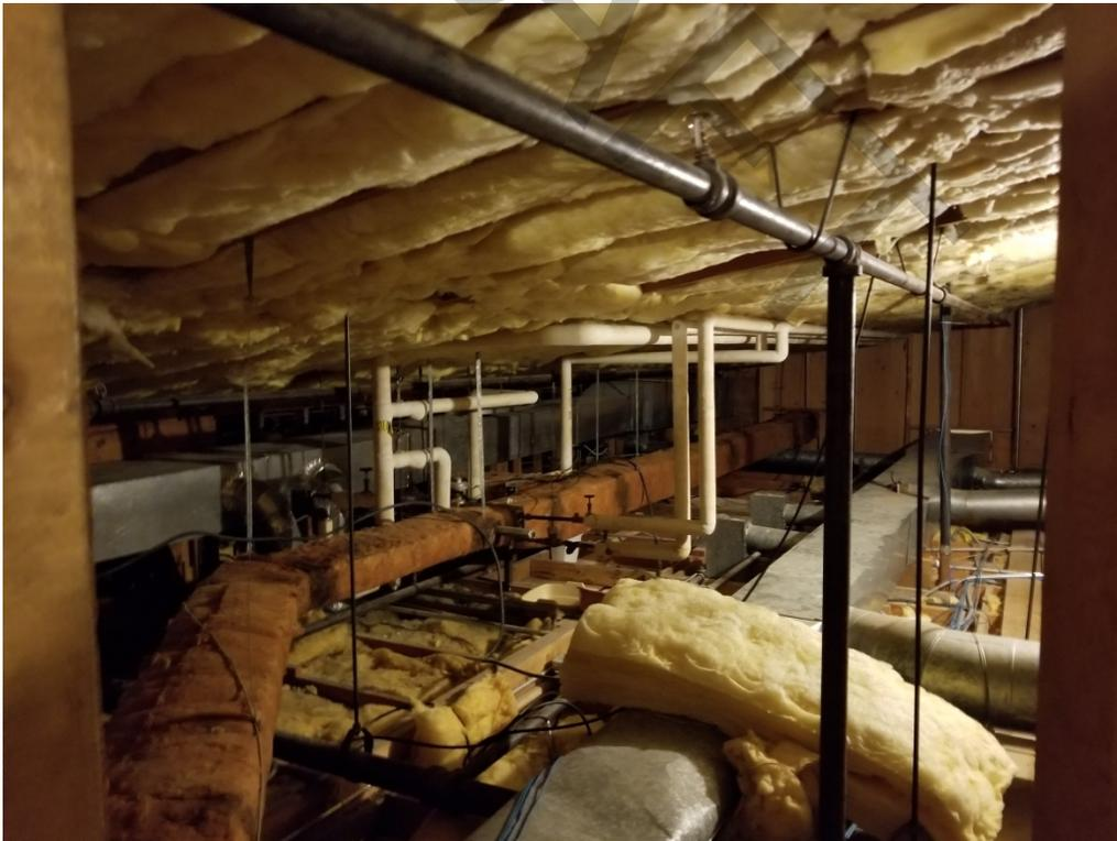
**Photo 14:** Presumed ACM TSI in the attic under the roof of the original building. (May 22, 2018)
