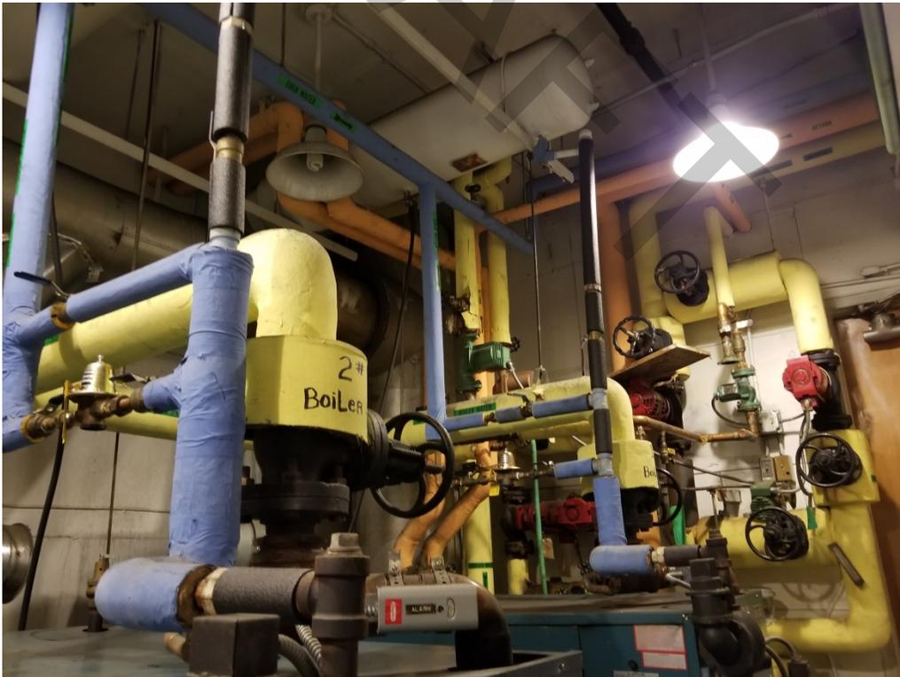
**Photo 12:** Presumed ACM TSI in the boiler room. Flue in back corner is assumed to contain ACM insulation. (May 22, 2018)
