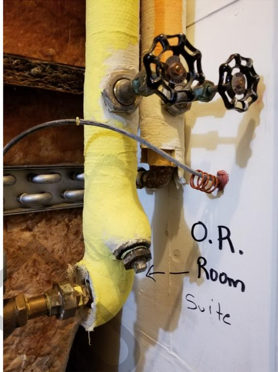
**Photo 15:** Exposed ends of presumed ACM TSI hard insulated joints. (May 22, 2018)
