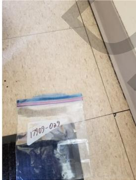
**Photo 6:** Off-white floor tiles in the stairway were ACM, and had a black mastic with trace amounts of asbestos. (May 22, 2018)
