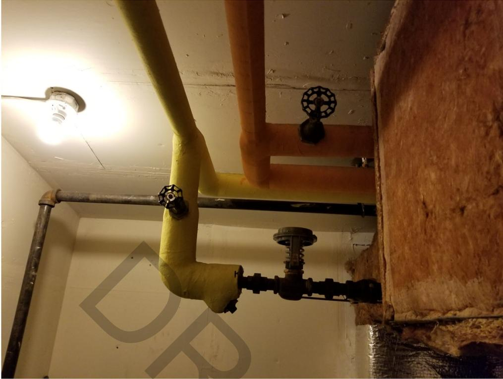
**Photo 13:** Presumed ACM TSI in the air handler room. Orange duct insulation on the right is not ACM. (May 22, 2018)
