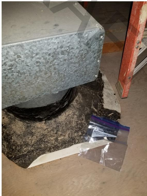
**Photo 2:** Tar paper skirts around penetrations in the new portion of the attic are ACM. (May 23, 2018)
