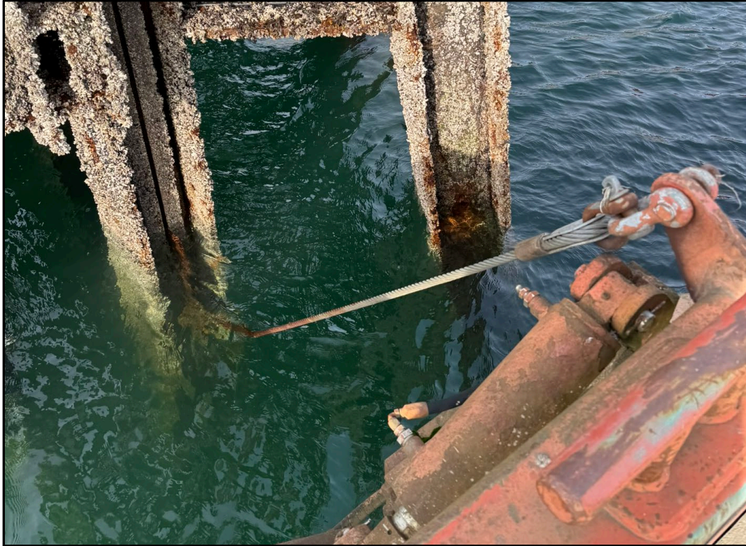
FIGURE 6. Tether cable on north side of barge ramp.
