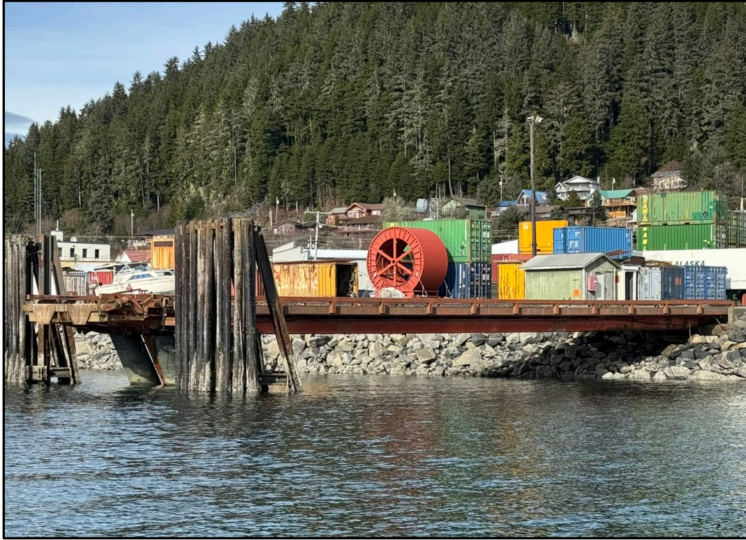
FIGURE 1. Overall view (south side looking north) of barge ramp.
