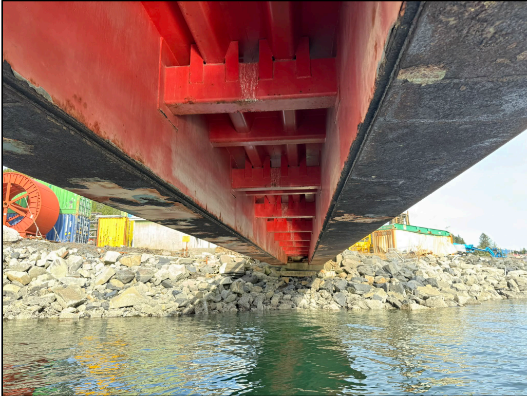
FIGURE 8. Bottom flange of barge ramp girders, looking shoreward from floatation tank.
