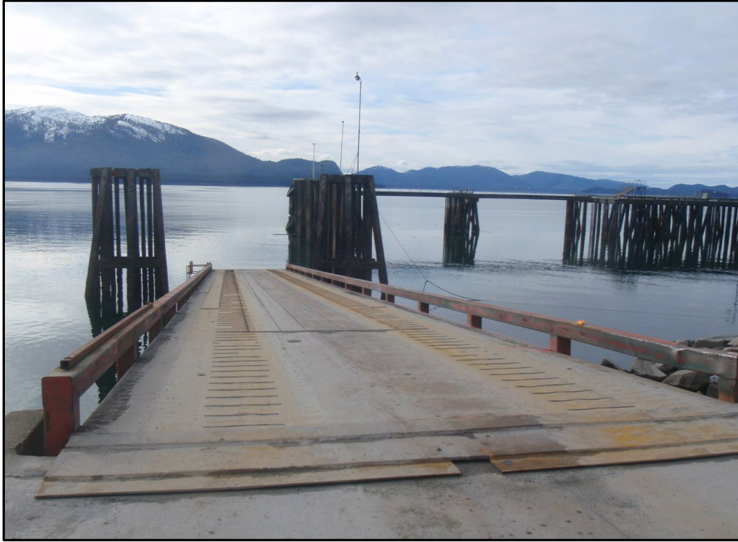
FIGURE 3. Barge ramp deck looking ramp from abutment.
