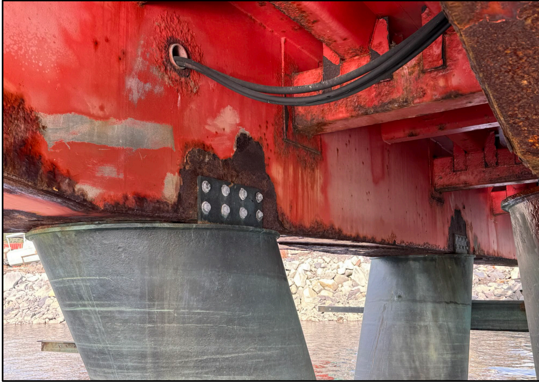
FIGURE 5. Flotation tank connection plates with new bolts.
