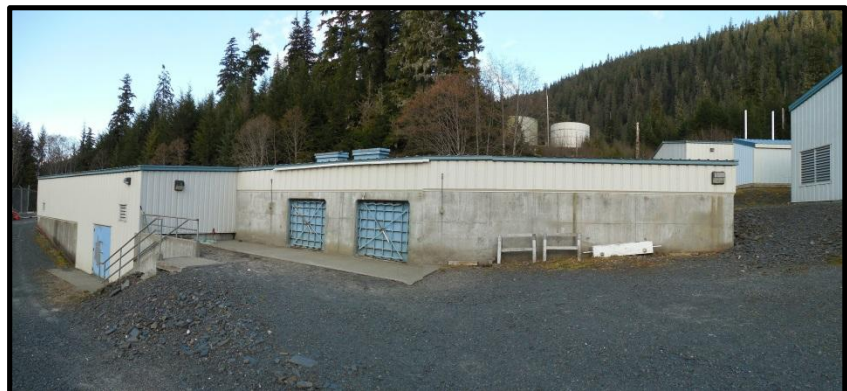
Photo 2 Water Treatment Plant
